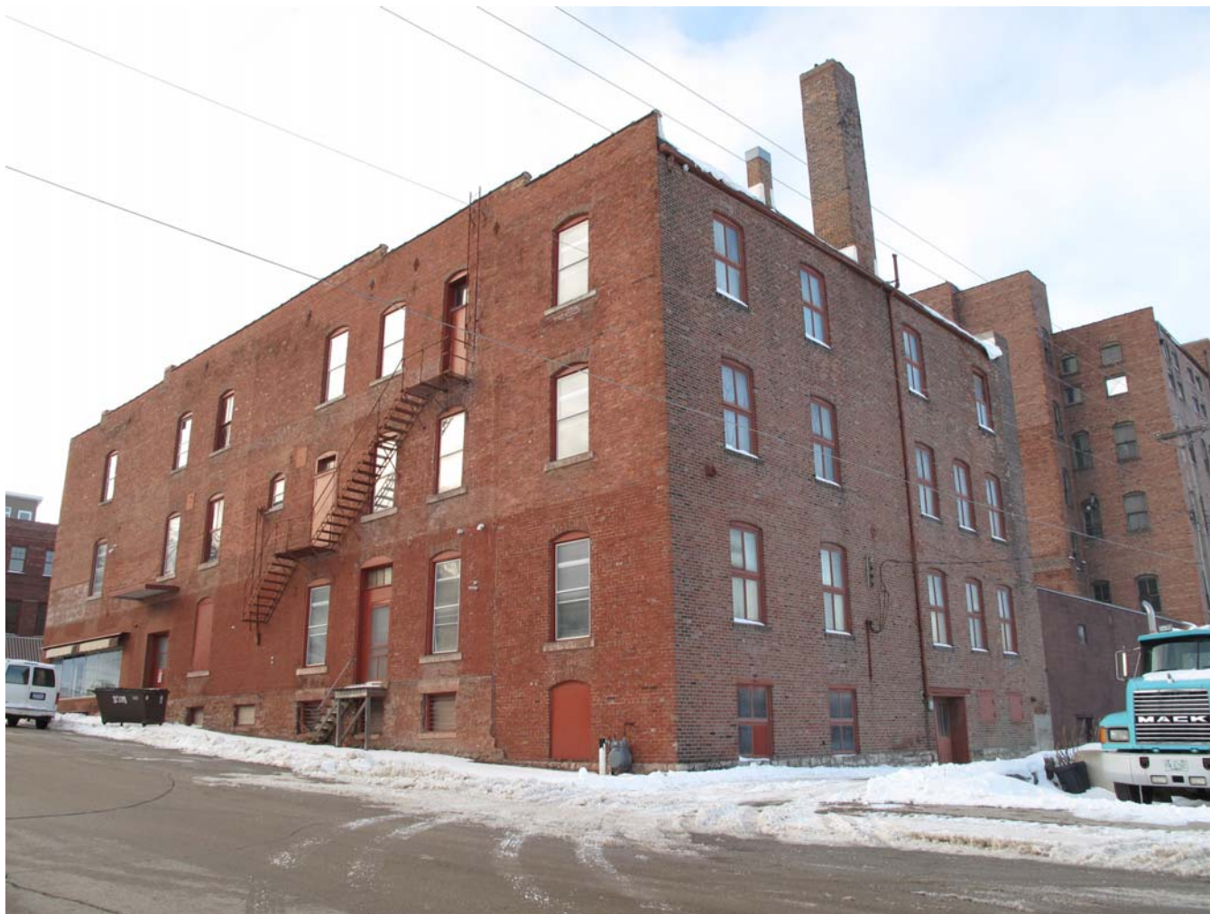
Building, looking northwest January 12, 2010 R.L. McCarley
