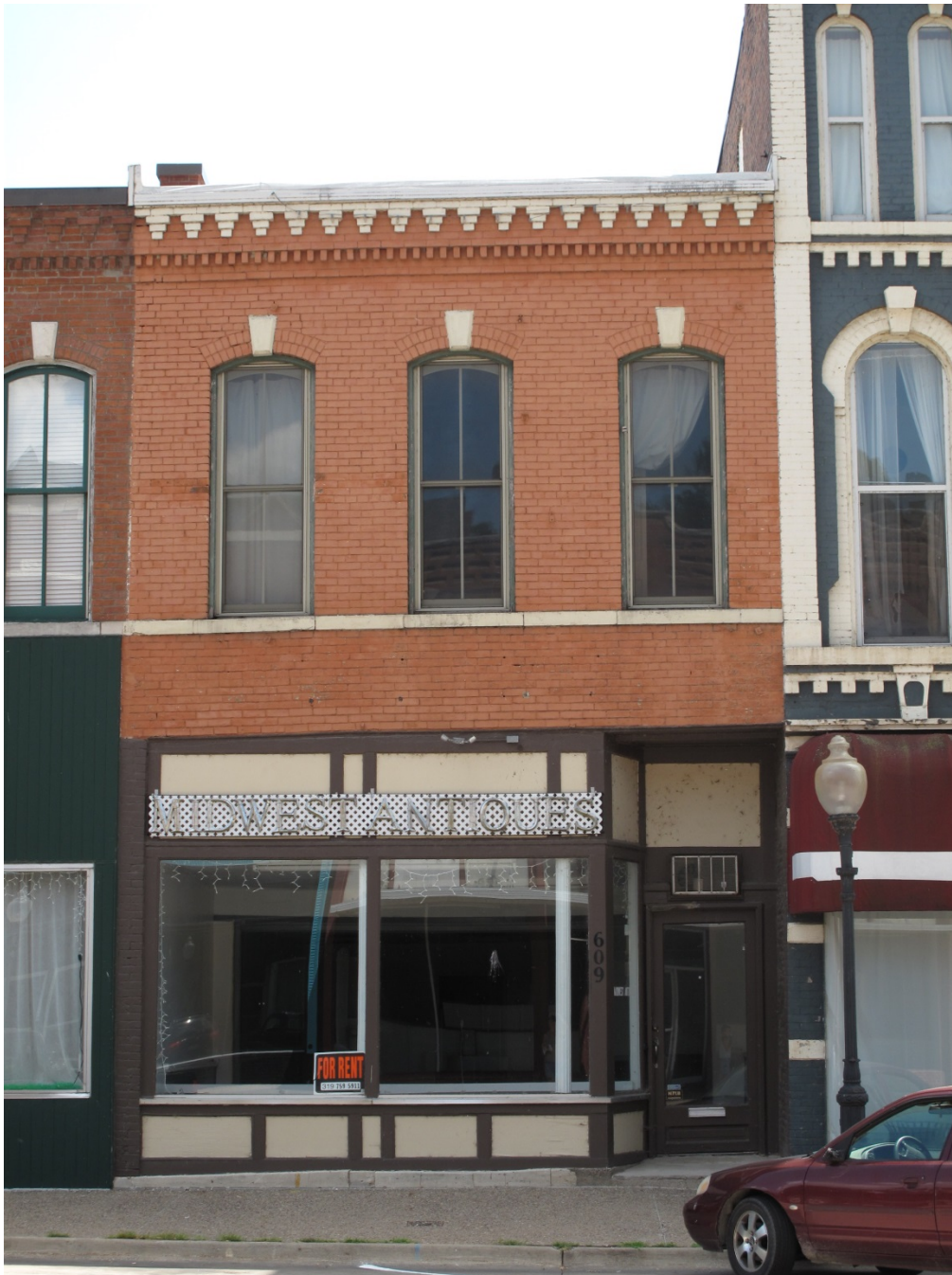
Photograph 29-01124-001 – North elevation, looking south (McCarley, July 17, 2013).
