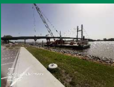
Piles for future dock being installed
