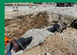
Forcemain Installation on Main Street
