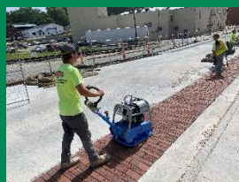
Jefferson Street paving near the Railroad Tracks
