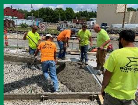
Jefferson Street paving near the Railroad Tracks
