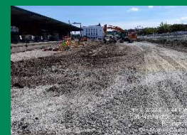
Grading work near the Port Building
