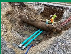
Sanitary Sewer Service construction on Main Street
