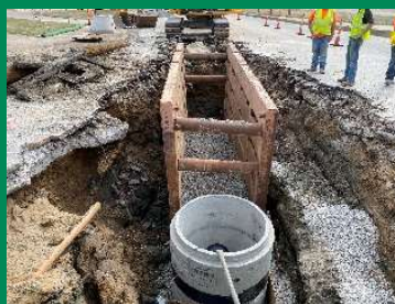
Sanitary Sewer Installation on Main Street
