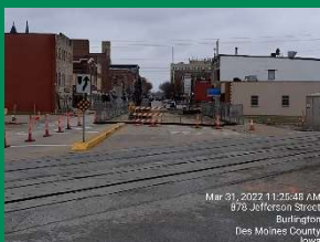
Jefferson Street Concrete Removal – Between 7 th & 8 th
