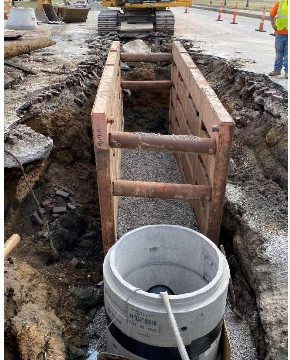
Sanitary Sewer Installation on Main Street
