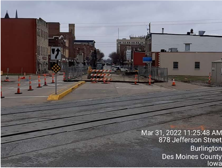
Jefferson Street Concrete Removal – Between 7 th & 8 th Street
