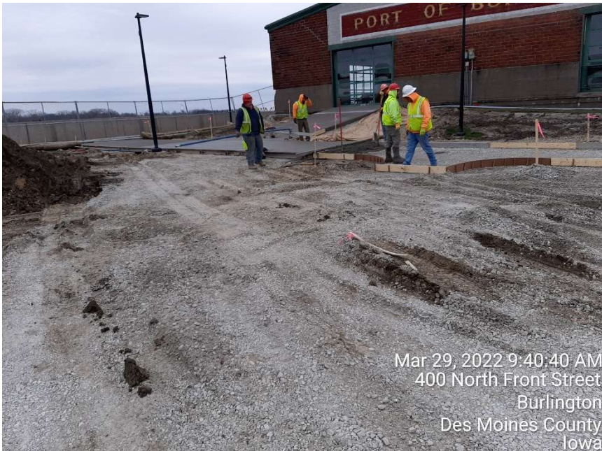
Sidewalk Paving near Port Building
