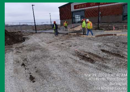
Sidewalk Paving near Port Building
