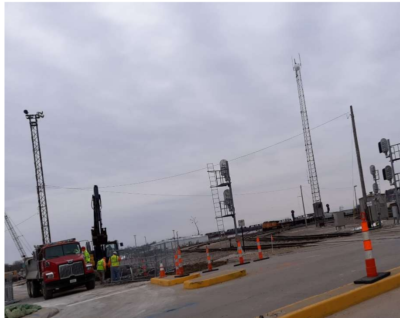
Pavement Removal at Market and Main Street
