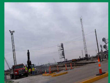
Pavement Removal at Market and Main Street
