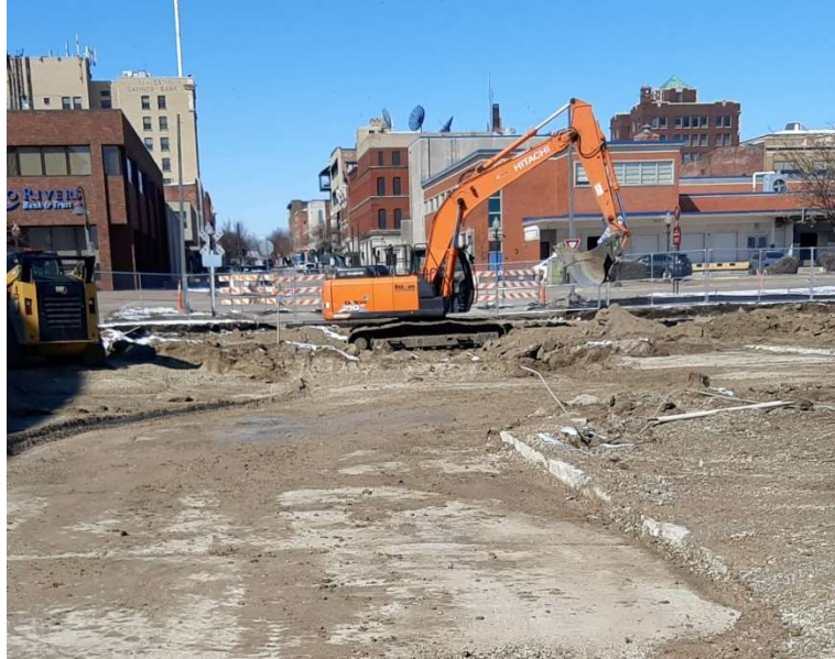
Utility work at Jefferson entrance in front of the auditorium.
