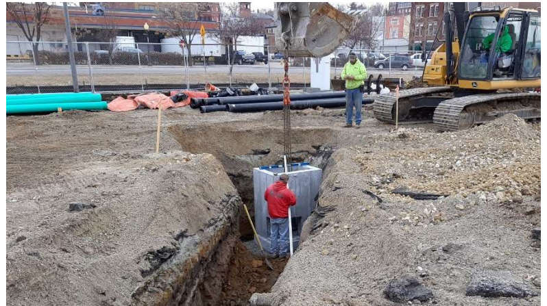
Storm sewer installation in front of the auditorium
