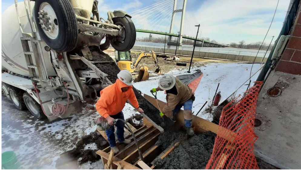
Stair construction on the North side of the Port Building
