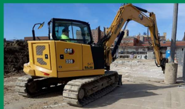
Parking lot pavement removal near the auditorium
