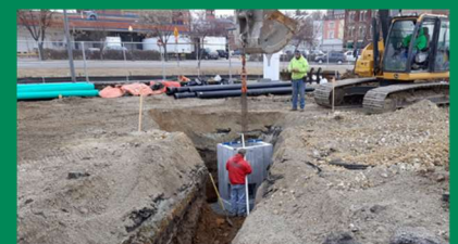
Storm sewer installation in front of the auditorium
