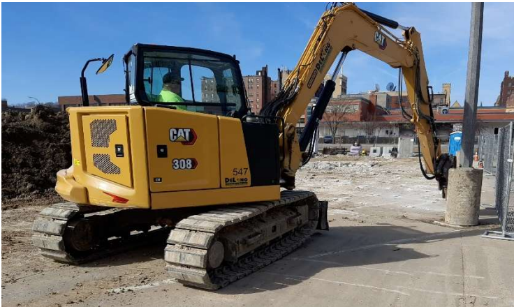
Parking lot pavement removal near the auditorium
