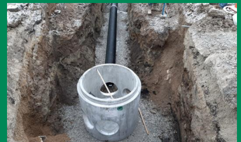
Storm sewer installation on north side of port building
