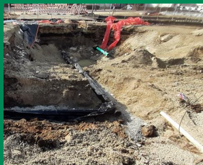
Watermain installation at Jefferson Street parking lot entrance
