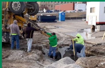
Storm sewer installation on north side of Port building
