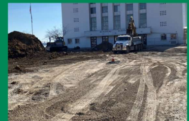
Construction of parking lot in front of the auditorium
