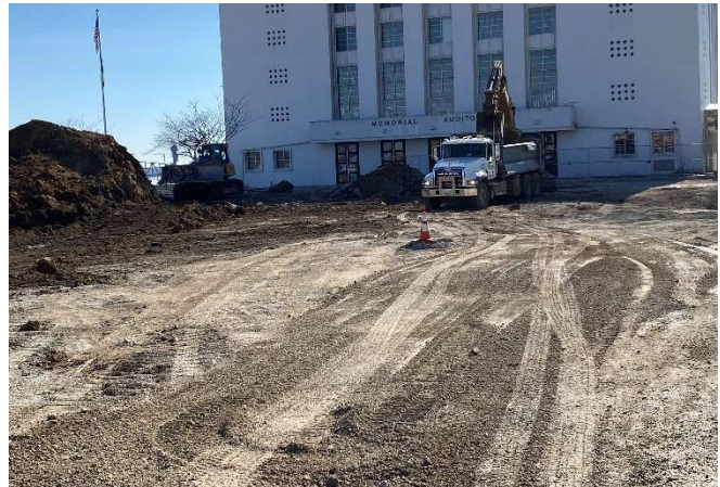
Construction of parking lot in front of the auditorium
