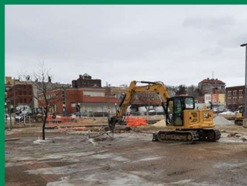
Pavement removal south side of parking lot
