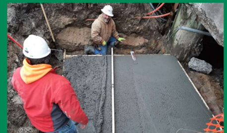
Concrete work on north side of Port building
