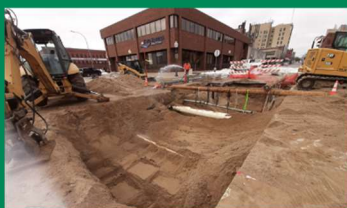
Water main and sanitary sewer installation and backfill
