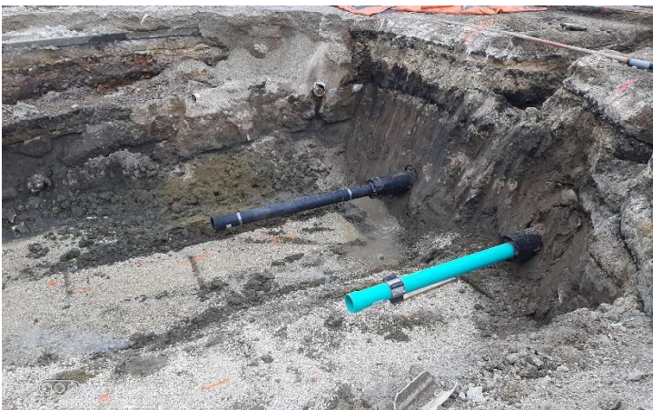
Watermain and sanitary sewer installation.
