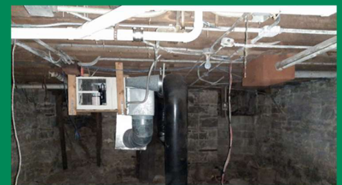
Basement inspections for Jefferson and Main project.
