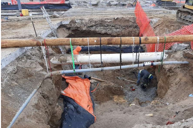
Water main and sanitary sewer installation in parking lot.
