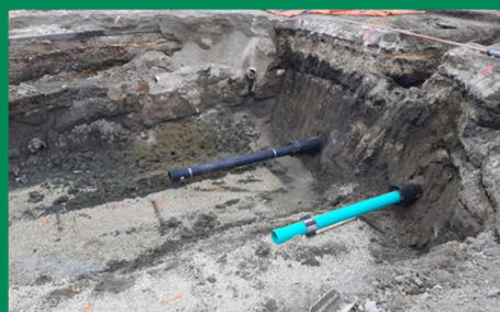
Watermain and sanitary sewer installation.
