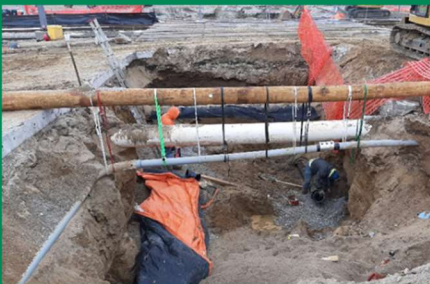
Water main and sanitary sewer installation in the parking lot.
