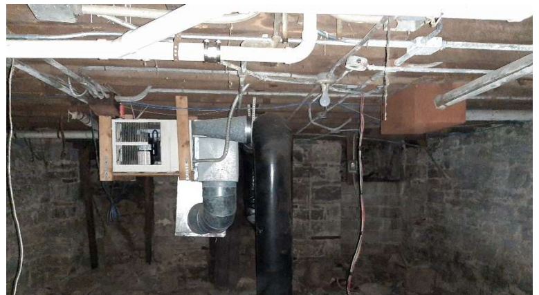
Basement inspections for Jefferson and Main project.
