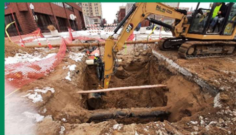
Excavation for watermain and sanitary sewer installation.
