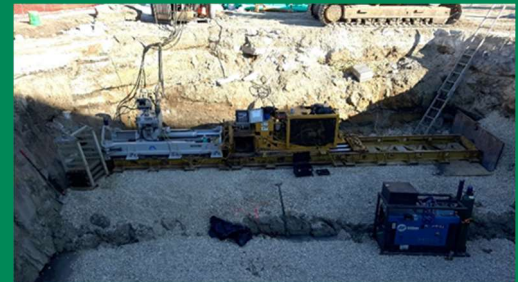
Watermain and sanitary sewer trench backfill installation and compaction.
