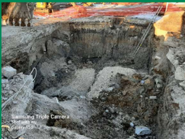
Boring preparation in parking lot for water main and sanitary sewer
