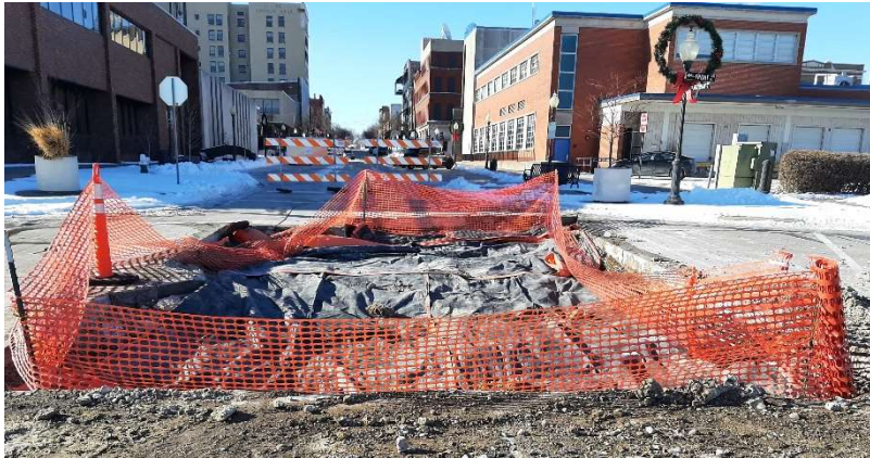
Boring preparation in parking lot for water main and sanitary sewer.
