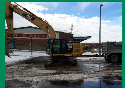
Parking lot construction on North side of Port Building.
