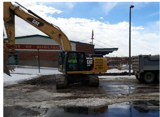
Parking lot construction on North side of Port Building.
