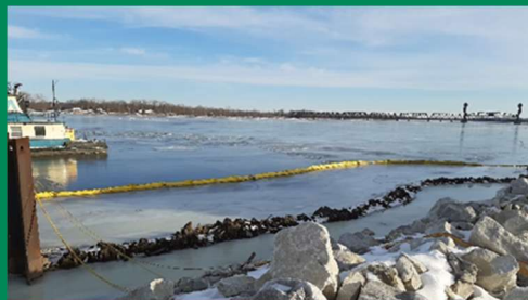
Boat ramp construction riprap installation.
