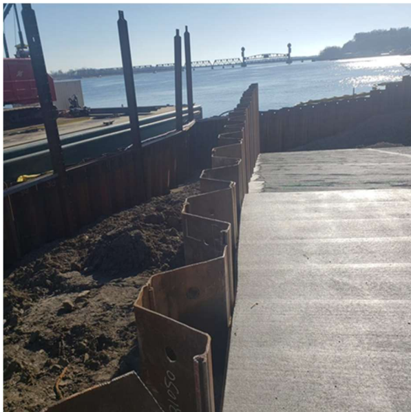
Boat ramp construction and jetty wall
