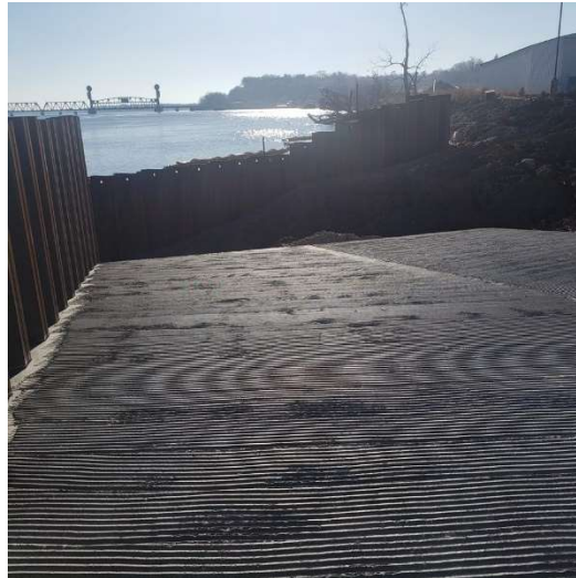
Boat ramp construction and jetty wall
