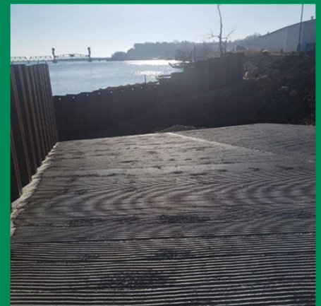
Boat ramp construction and jetty wall
