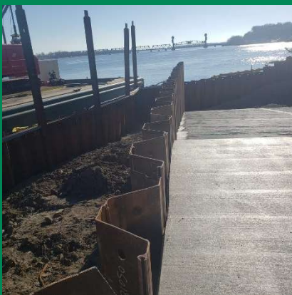
Boat ramp construction and jetty wall
