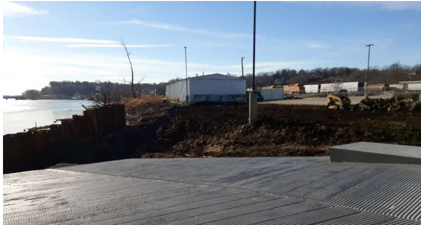
Boat ramp construction and grading
