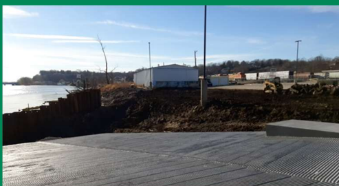
Boat ramp construction and grading
