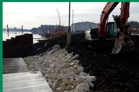
Rip rap installation along boat ramp
