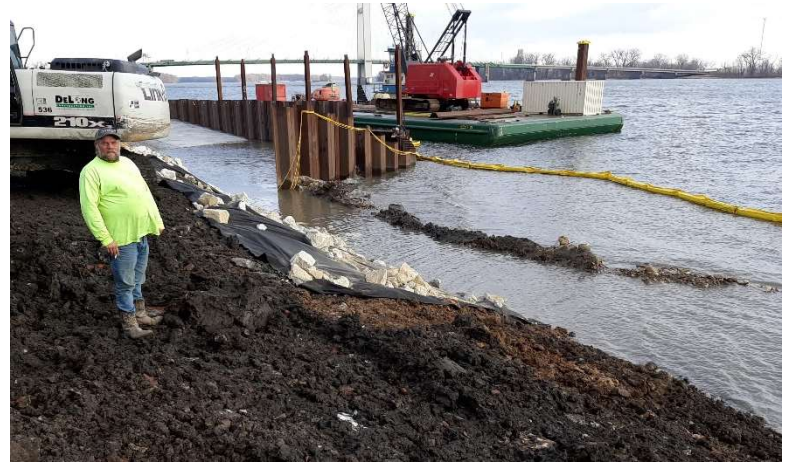
Boat ramp, jetty wall, and rip rap installation along river side.
