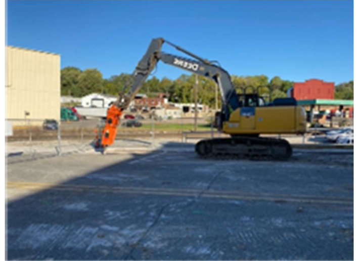
Pavement Removal Jefferson
