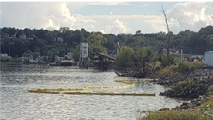
Silt Curtain installed as part of Pollution Prevention Plans
