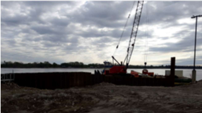
Coffer Dam Construction
