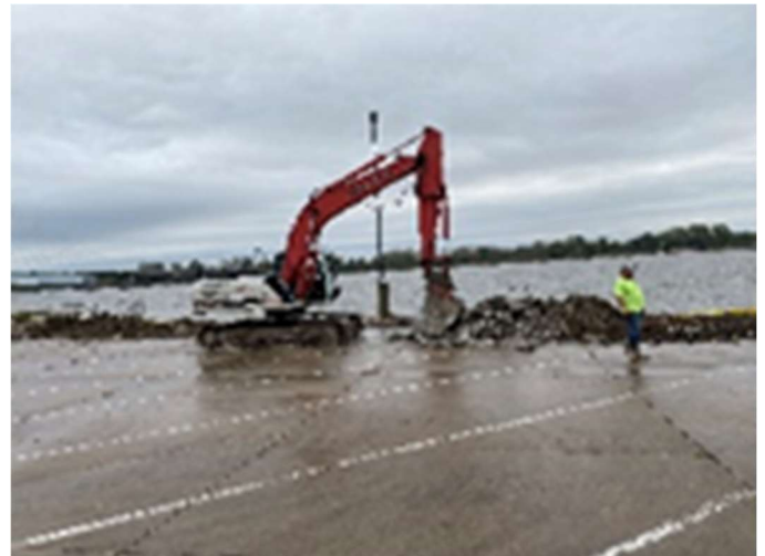
Pavement Removal Riverfront
