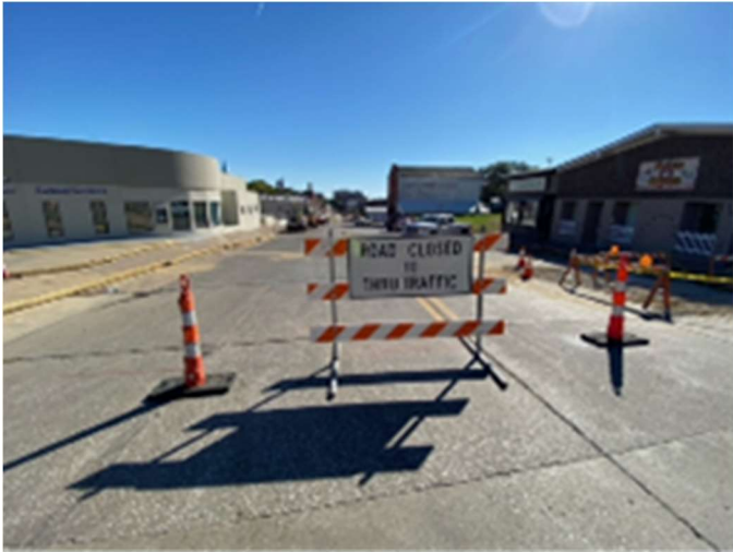
Jefferson Road Closure
