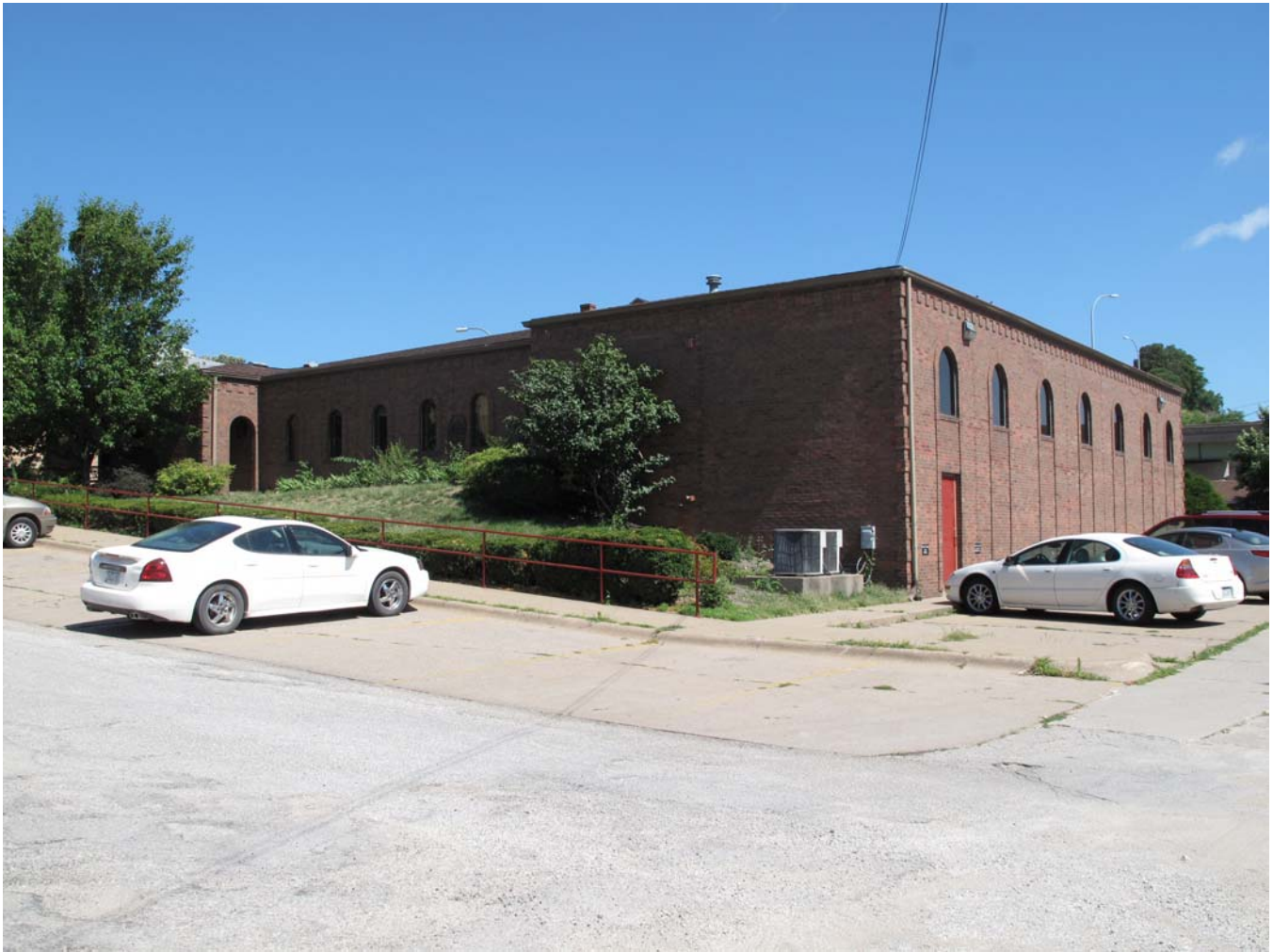
Photograph 29-03666-002 – South and east (rear) elevations, looking northwest (McCarley, June 20, 2012).
