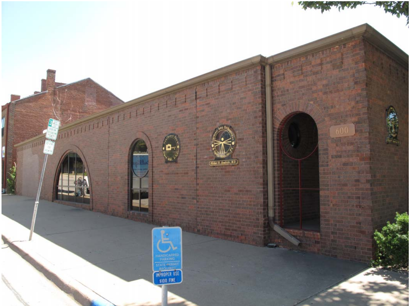
Photograph 29-03666-001 – West (front) elevation, looking northeast (McCarley, June 20, 2012).
